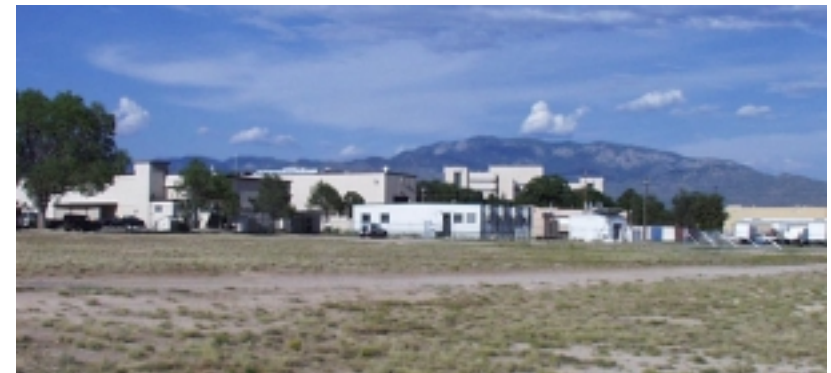
Electromagnetic Energy/RF Effects Laboratory
